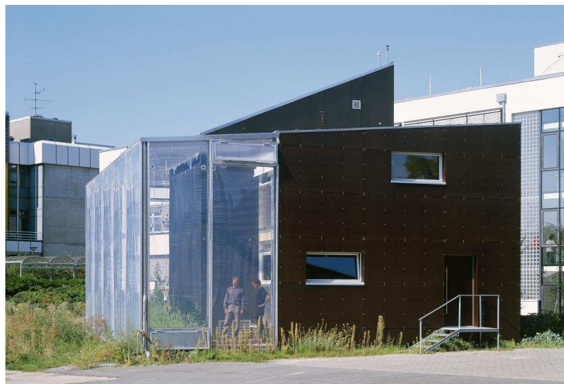
Figure 1: Demonstration building with integrated humid air solar collector system at the site of Technische Universitaet Berlin, Chair Building Technology and Design.
