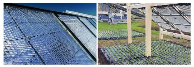
The transparent solar panels from Insolight (figure on the left) possess a micro-tracking technology with which light transmission can be adapted. Lamb's lettuce is grown under the modules at the Grüental campus in Wädenswil (figure on the right).
