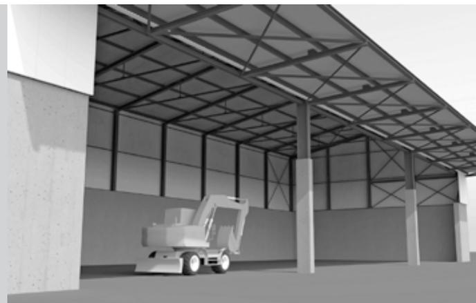
as snow can be moved by the wind and slide from the roof onto the canopy below. The snow and wind loads are carried by the girders, which are designed as trussed beams. Special attention was paid to the use of compact components and simple assembly.
