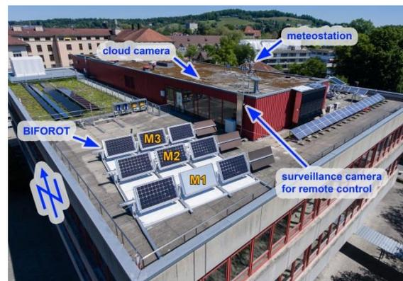
**Figure 2:** South orientated installation of the BIFOROT test array on the roof of the ZHAW in Winterthur. Aerial view on the roof and test array from southwest direction. The module tilt angle is changing permanently in a synchronized manner within an interval of one minute. Module 1 to module 3 (M1 –M3) are the devices under test (DUT).
