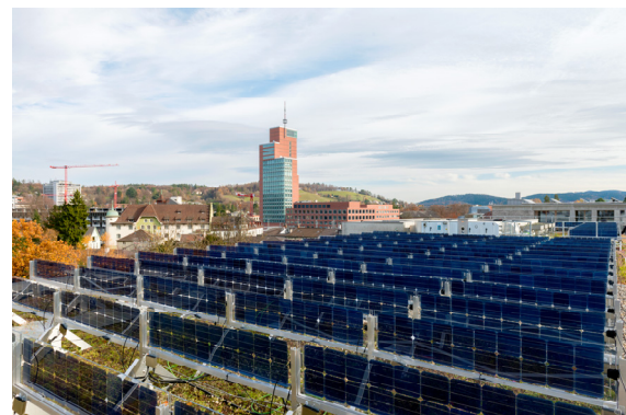
Figure 1 Vertically east-west mounted bifacial modules installed on the green roof in Winterthur, Switzerland with a rated output of 9.09 kWp. The east-west-facing modules have a tilt angle of 90° and an azimuth angle of -65° for the front side and 115° for the rear side. (used azimuth angle definition: east = -90°, south=0° and west = 90°)
