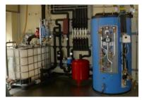
The entire configuration of the installation including the measurement points is shown in the **P&ID** (**Piping and Instrumentation Diagram**). The cooling circuit of the solar thermal facility also serves the ORC, which is also included in the P&ID. The measurement data is collected, recorded and visualized using a National Instruments data acquisition device with LabView visualization.
