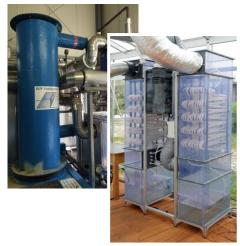
Figure 1: ZHAW and the project partner Watergy tested the absorption technology in previous projects: the High Temperature Condensing Technology, installed by Bergmann (ZHAW) recovers heat from the flue gas in an ab- /desorption process (top); an absorption box of Watergy is installed as air conditioner in a prototype building in (bottom)
