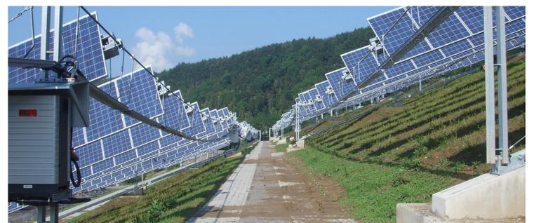
Fig. 1: One-axis tracking 650 kW, Lonza Solarpark, Germany
