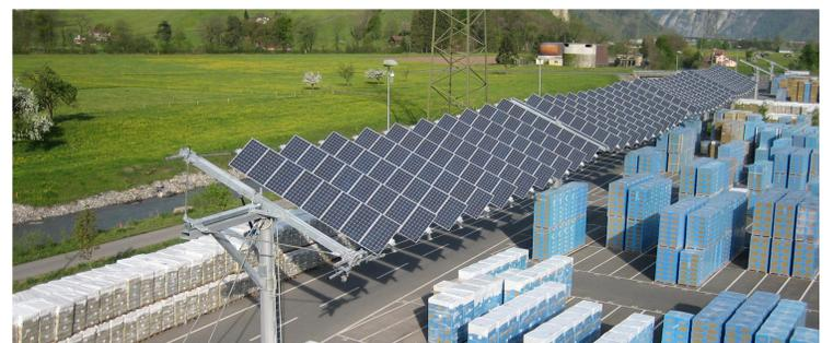
Fig. 2: Two-axis tracking 60 kW, Flumroc AG, Switzerland
